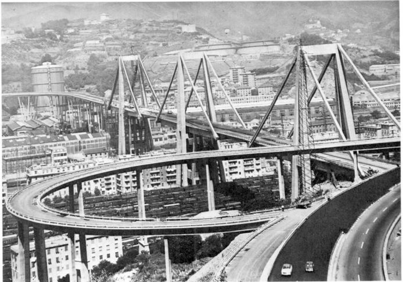
Figure 3 - General view of the structure.
