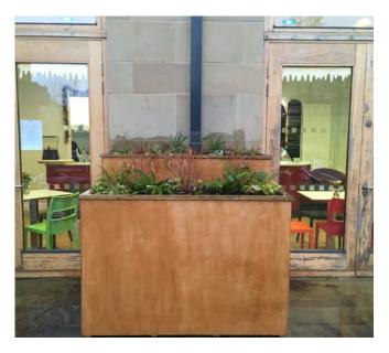
Rain garden planters are being installed in the courtyard of Hebden Bridge Town Hall to show how small interventions can be used to slow run-off and temporarily store water during storm events in our urban areas. The planters will intercept water from downpipes around the edges of the courtyard, providing water attenuation and biodiversity in an attractive way whilst maintaining the usability of the courtyard as a flexible open space.
