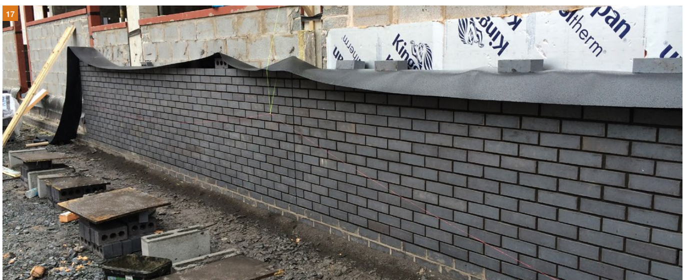
Protection from rainfall, note stacks of bricks also covered.
